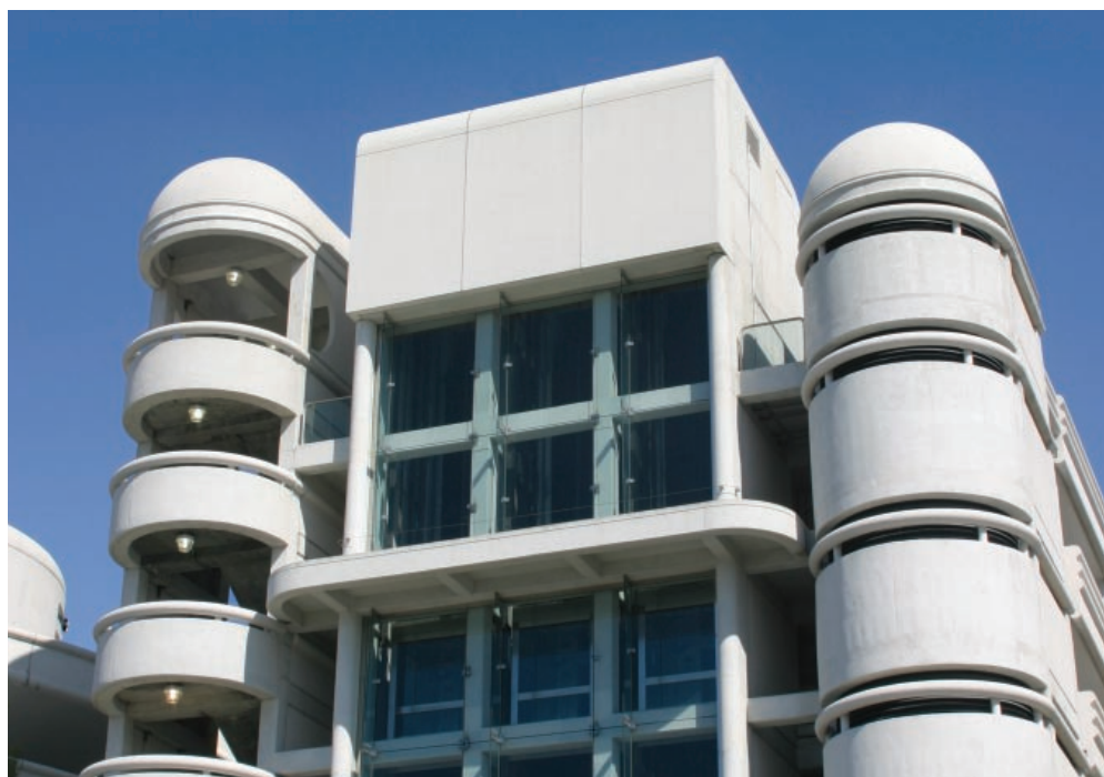
SFO's new Long-Term Parking facility.
